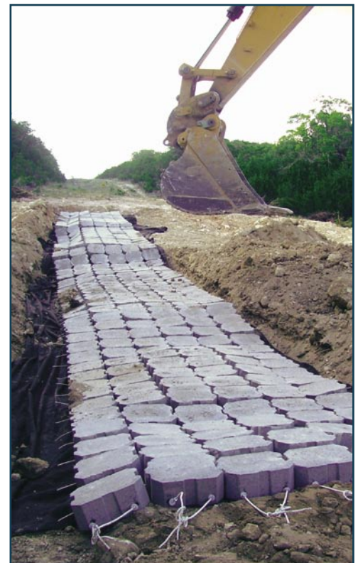
Mats being installed
