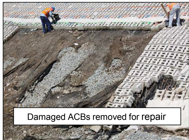
Figure 5. Photos Showing Damage to Bottom of ACB Armorment Following Overtopping of Portugués Cofferdam (Photos Courtesy of USACE)
